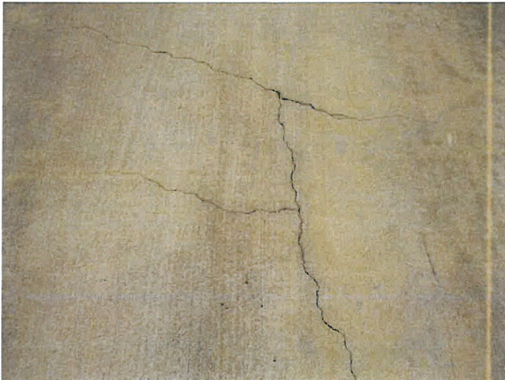
Cracking and Staining on Roof
