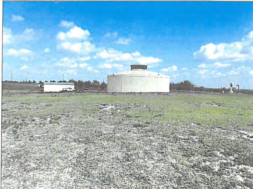
Figure C-2. Hickory Walk WTP Ground Storage Tank
