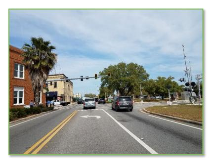
For the 1st Street streetscape project, CivilSurv prepared a traffic analysis to determine if the traffic signal at the intersection of 1st Street and Central Avenue was warranted or if the intersection could be converted from a traffic signal-controlled intersection to a 4-way stop to better conform with the streetscape project.
