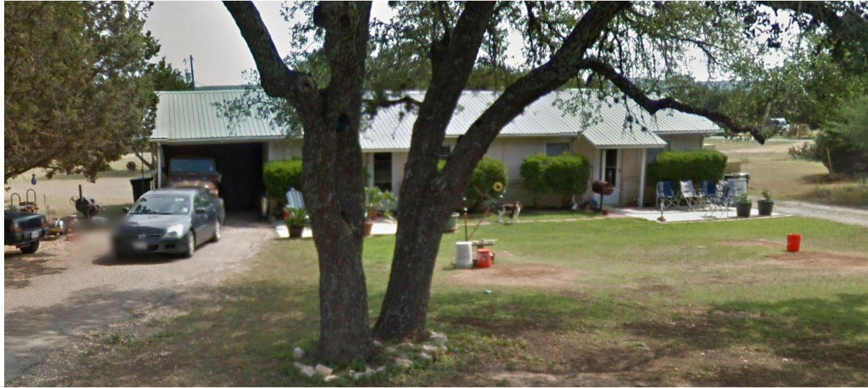
Exterior View of Existing Duplex
