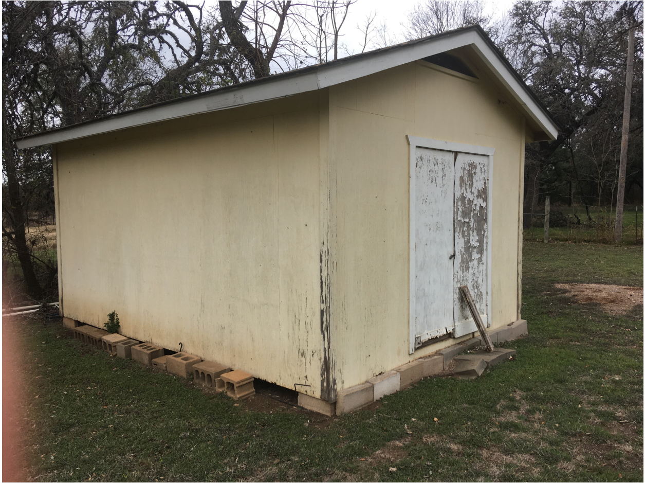
#301 Old Fitzhugh Rd. – Existing Shed:
