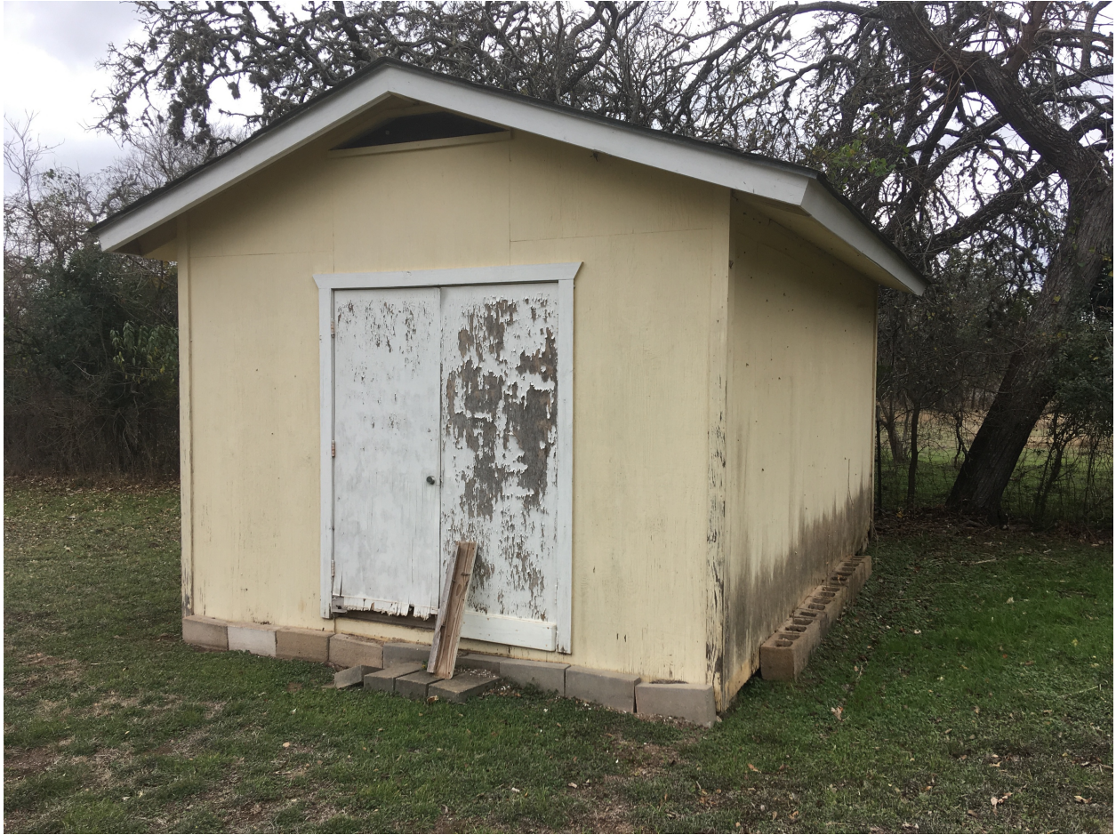
#301 Old Fitzhugh Rd. – Existing Shed:
