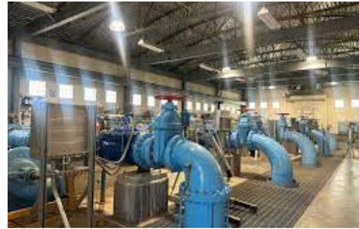
Figure #. West Travis County PUA Facility
