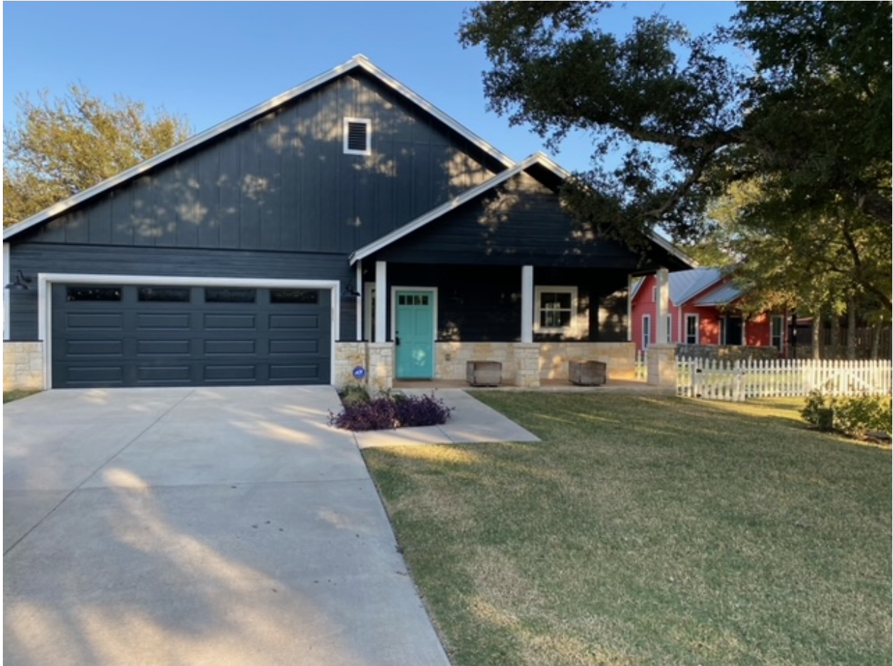
#231 Haydon Lane: “Current Color” –Front of Property. COA Application Photo- 11/4/21 (SW # 6992 Inkwell)
