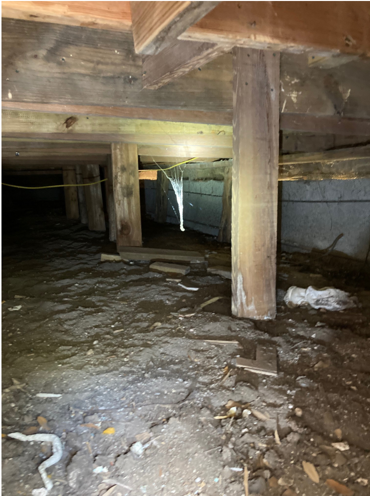
Severe damage to cedar piles - full replacement and leveling required
