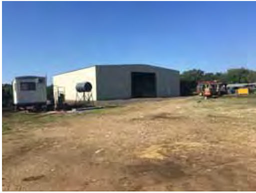
Exterior - Existing Barn - HCLE Owned
