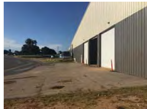
Event Center - East Entry to Staging Area
