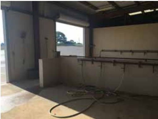
Event Center - Wash Down Area
