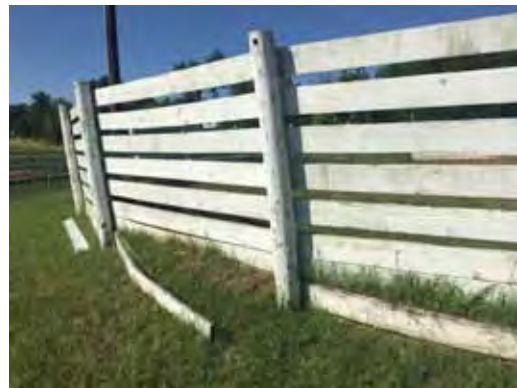
Exterior- Round Pen - Under Construction
