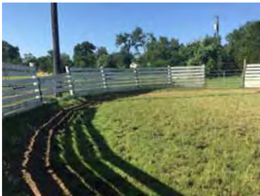
Exterior- Round Pen-Under Construction
