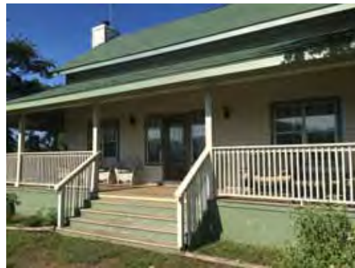
Exterior - Existing House
