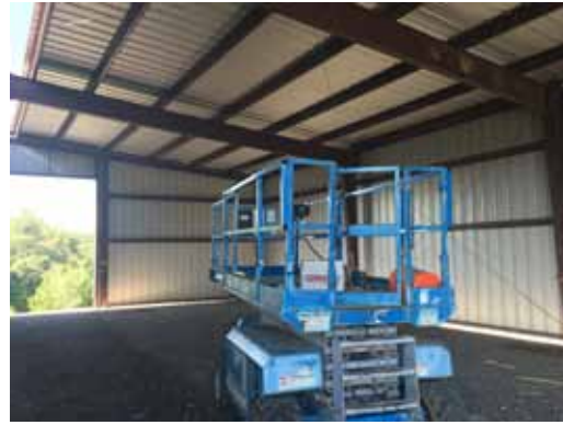
Exterior- Existing Barn (Interior) - HCLE Owned
