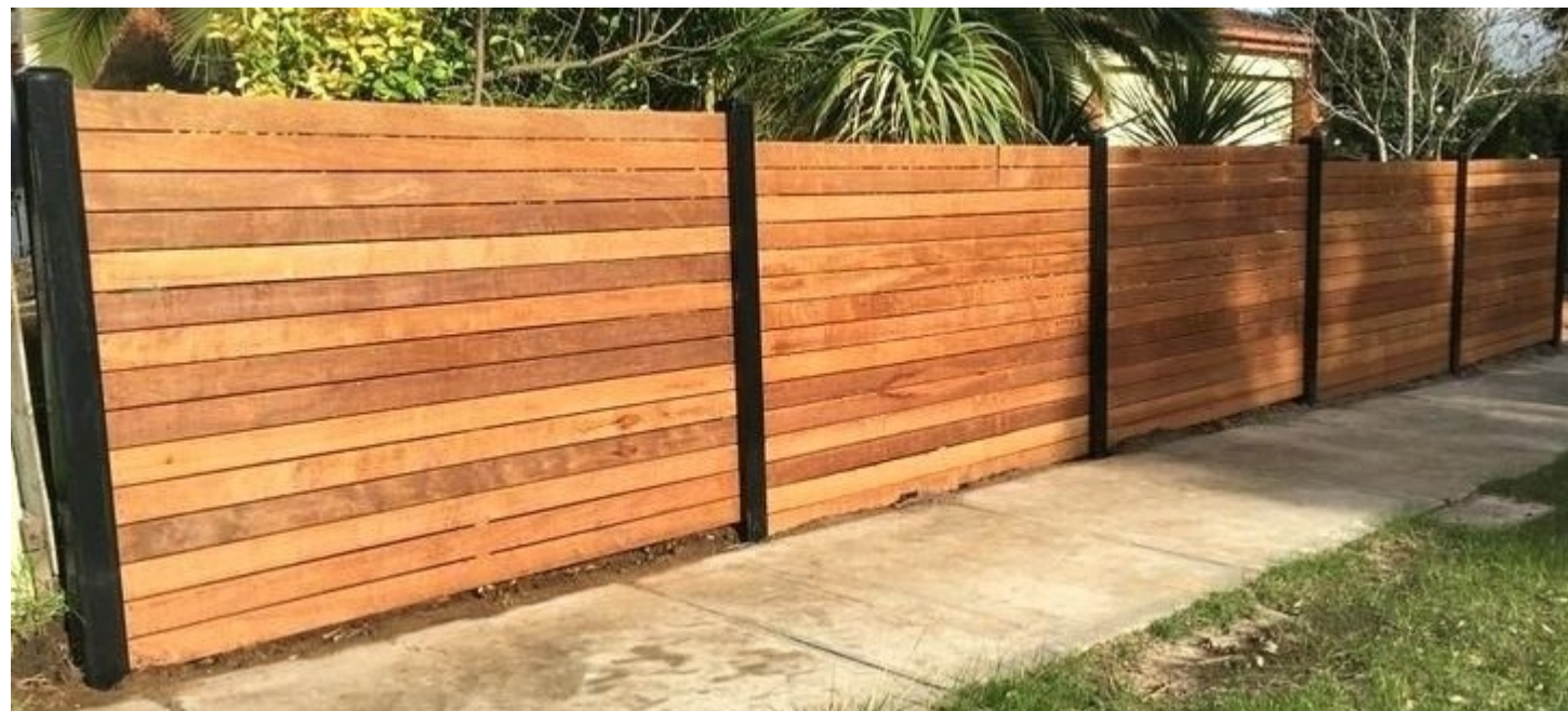
Stained 2X6 S4S Cedar Plank Screen Panels installed between 4X4 Steel Porch Posts and 4X6 Steel Porch Beams (All Steel to be painted Black)
