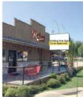
New Wall Sign - Day
