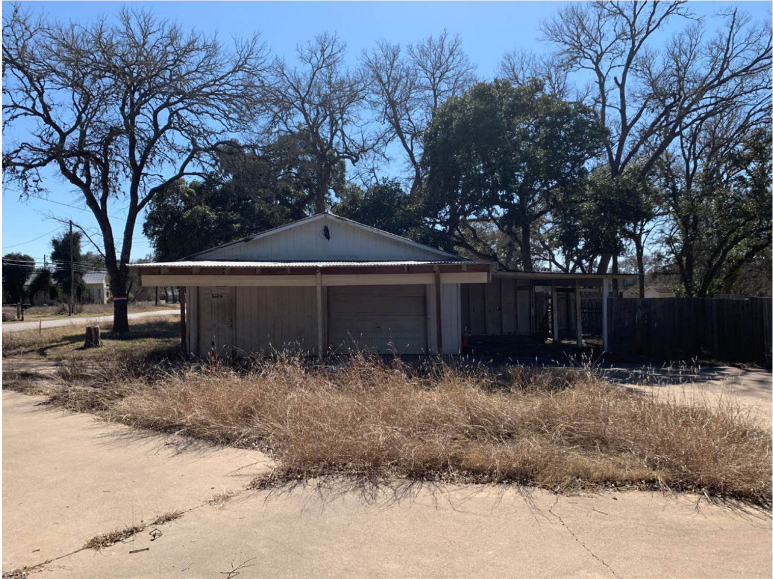
Existing garage to be removed.
