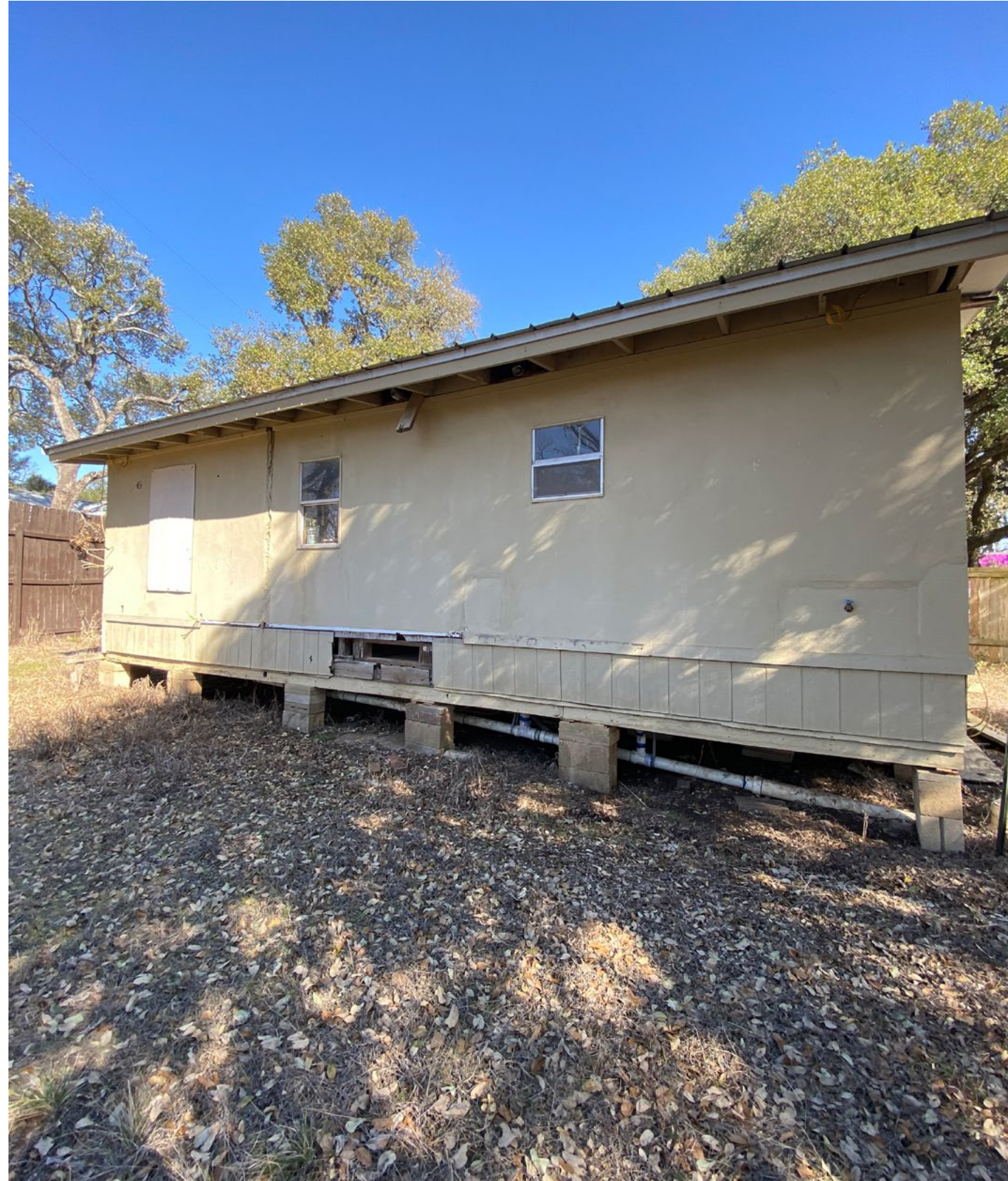
Non-contributing addition to existing homestead, to be removed.
