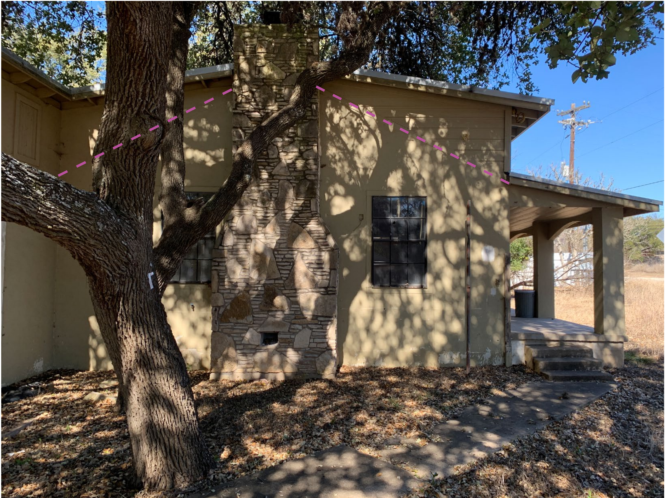
Existing homestead – propose restoration of original gable roof profile
