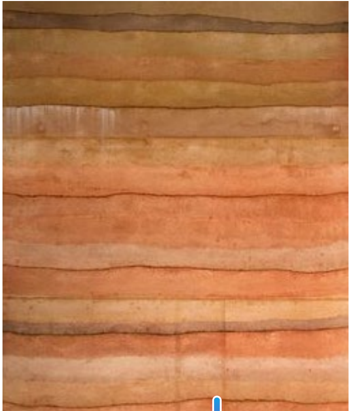
Rammed earth accent wall
