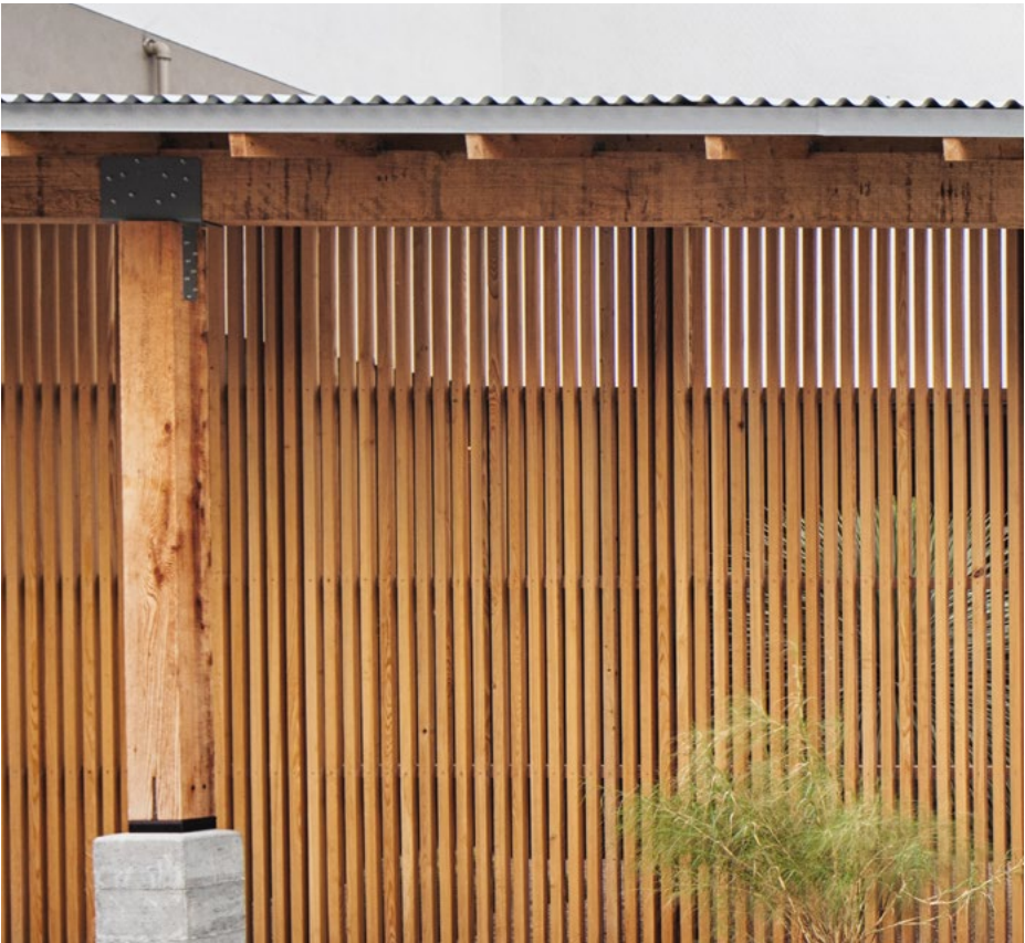
Cypress framed porch.
