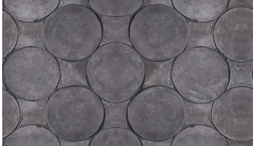
Extruded cement tile @ patio
