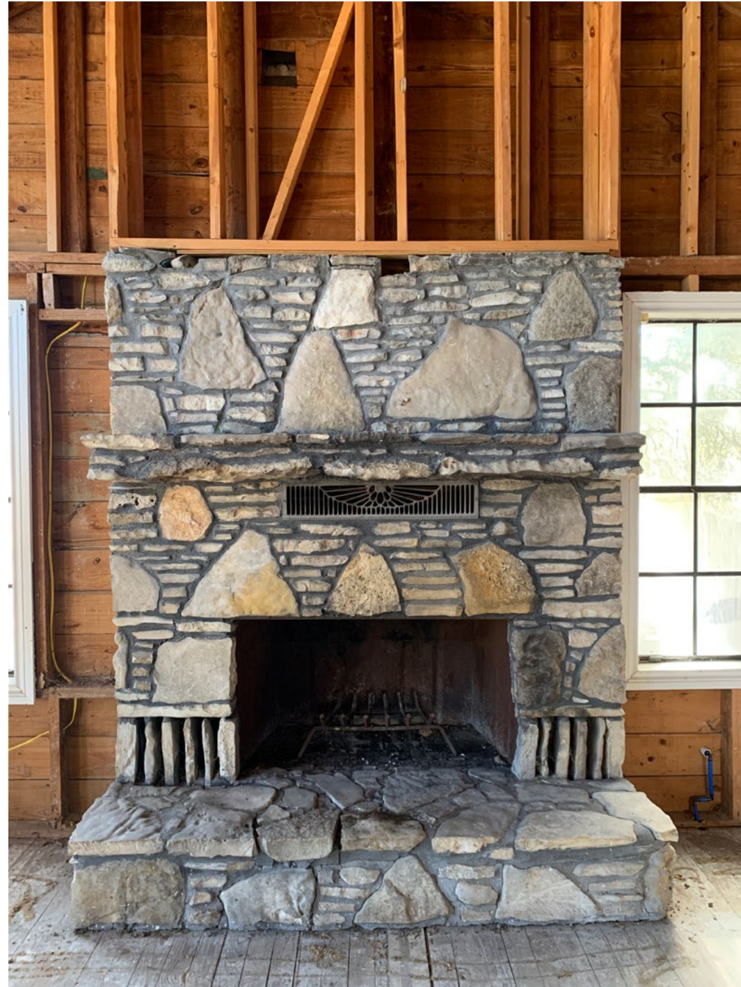
View of fireplace from inside existing homestead. Existing fireplace to remain.
