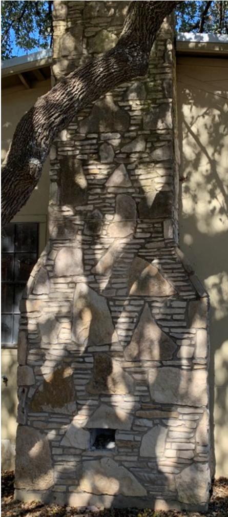
Existing masonry chimney
