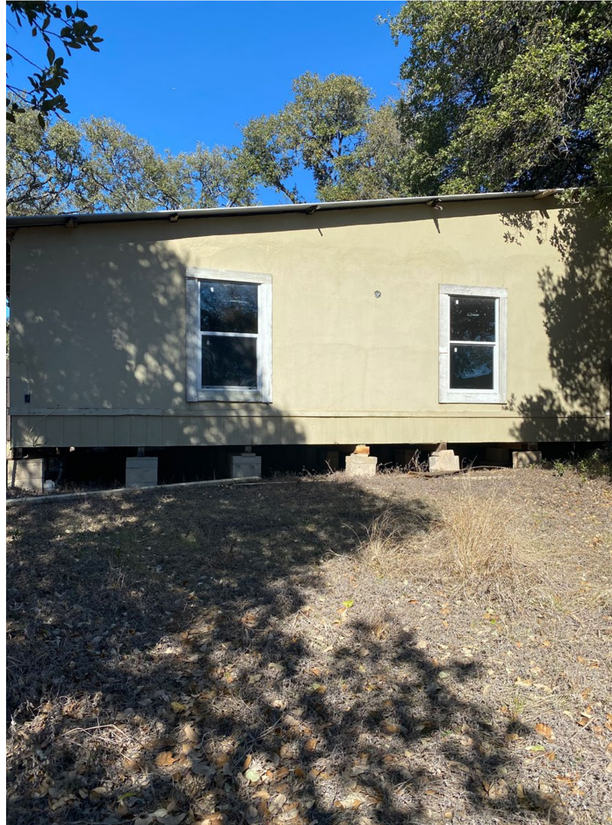
Non-contributing addition to existing homestead, to be removed.
