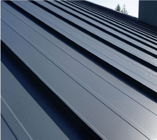
Standing seam metal roof.
