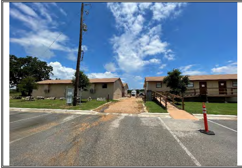
Modular buildings in area of acquisition
