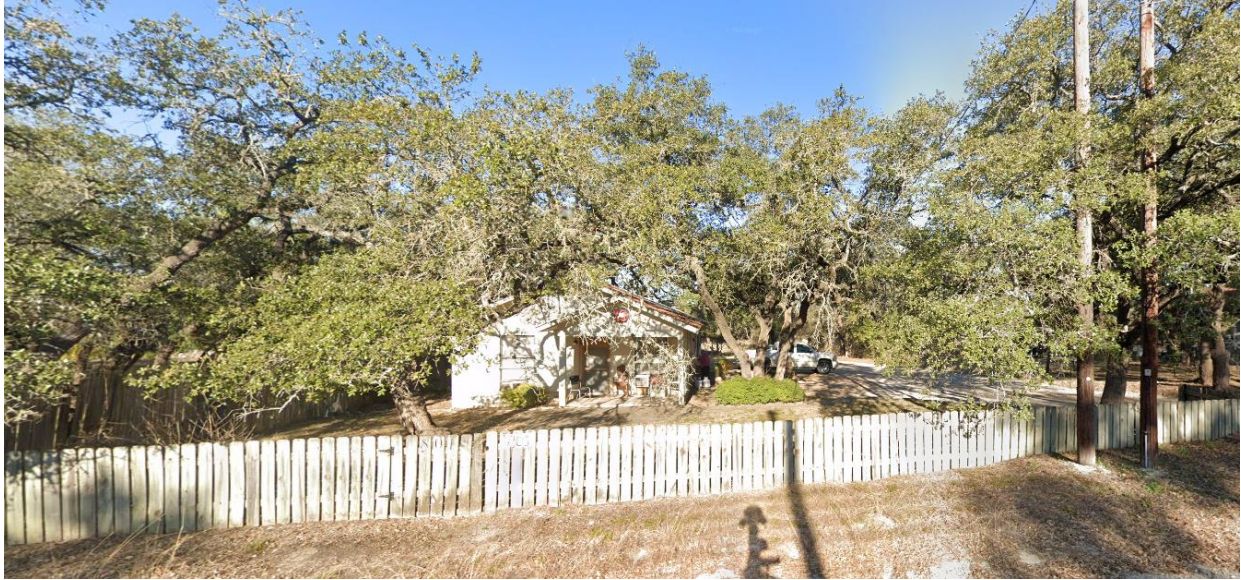
801 OFR: Current Condition. Image from Google Maps, March 2022.
