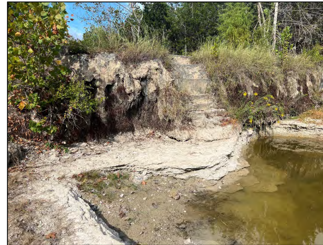
Photo 8: Stairs leading to top of historic dam.
