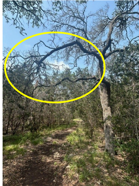
Photo 11. Dead branches over walkways should be removed.
