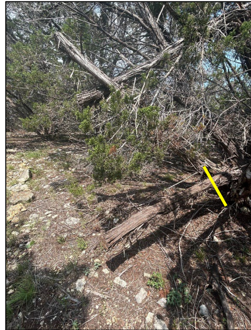
Photo 5. An old stub cut that was found at the site. The proper cut should be made at the yellow line where the stub meets the live stem.
