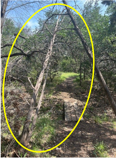
Photo 10. Dead trees over walkways should be removed.
