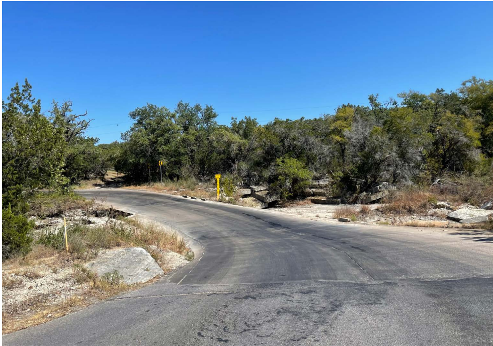
Figure 14. Bell Springs Rd
