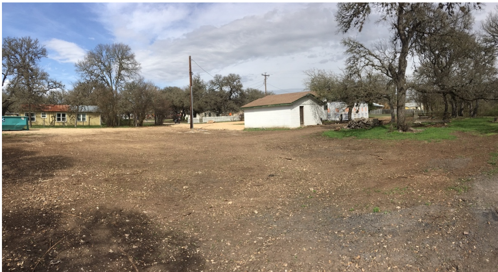
#264 South College St. –Rear View of Property w/Site Work Underway: Photo 3/14/21
