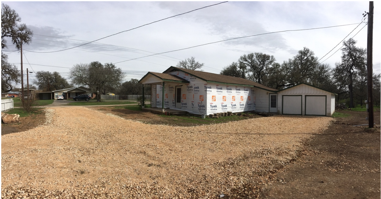
#264 South College St. –Front of Property w/Exterior Rehabilitation Underway:
