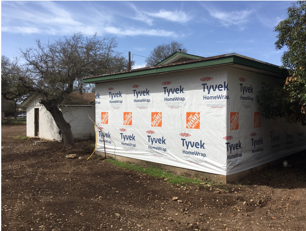
#264 South College St. –Rear of Dwelling & Garage w/Rehabilitation Underway: Photo 3/14/21
