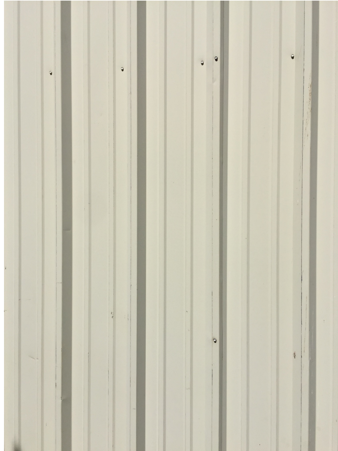
Tan Colored Metal Wall "R" Panels to match Existing Metal Wall "R" Panels
