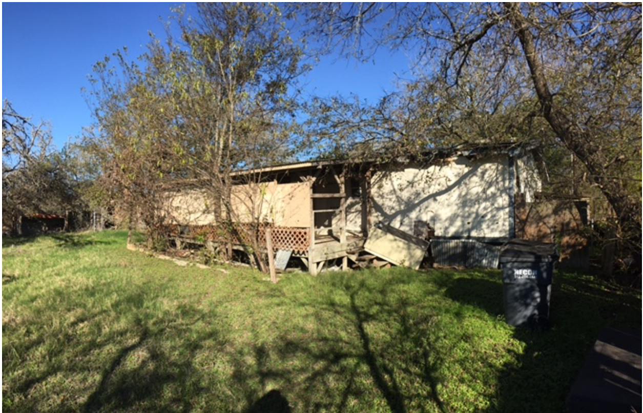
Existing Mobile Home / OFR Frontage / 28491 RR-12 / November 28, 2021
