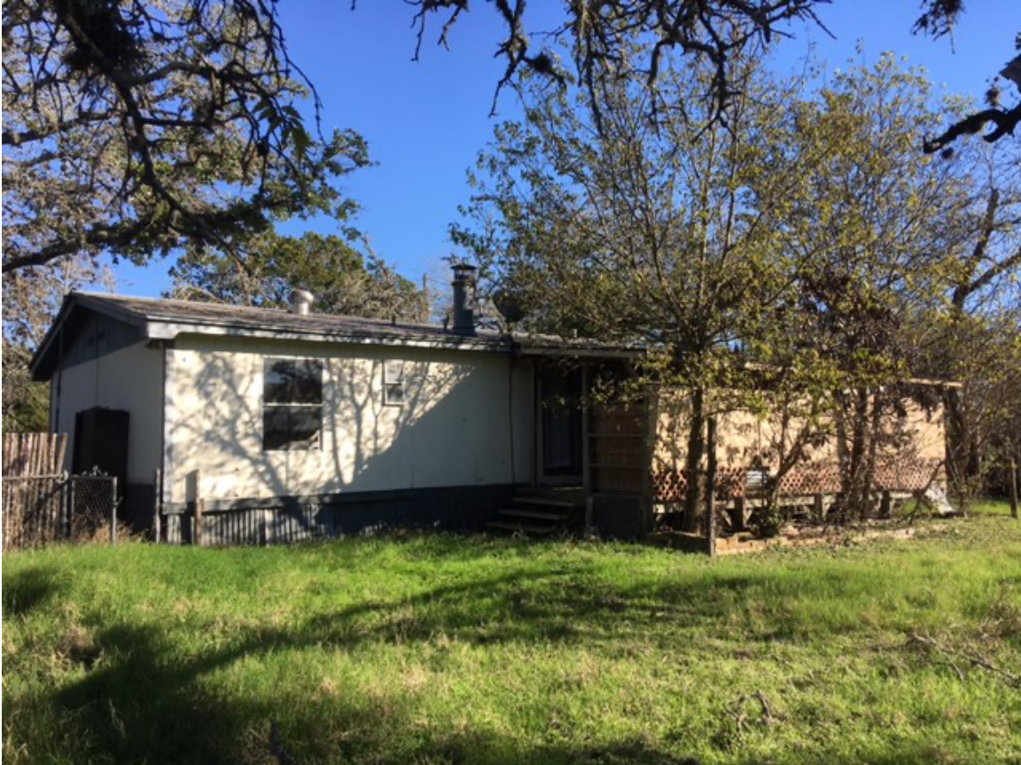
Existing Mobile Home / OFR Frontage / 28491 RR-12 / November 28, 2021
