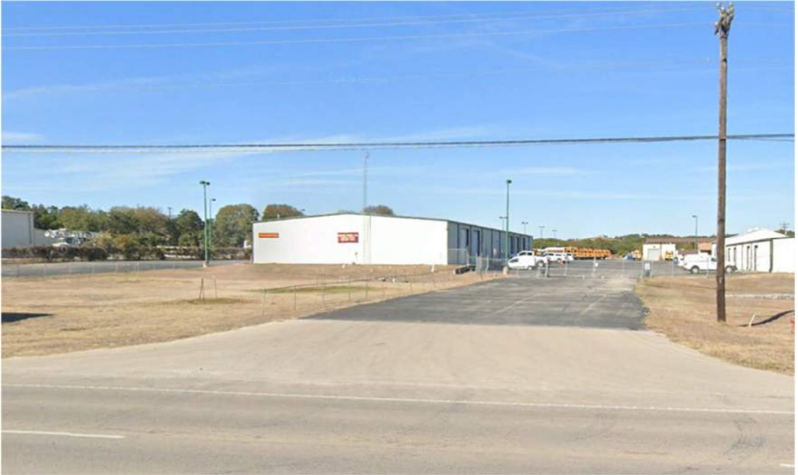
Looking at Southbound DSISD Driveway
