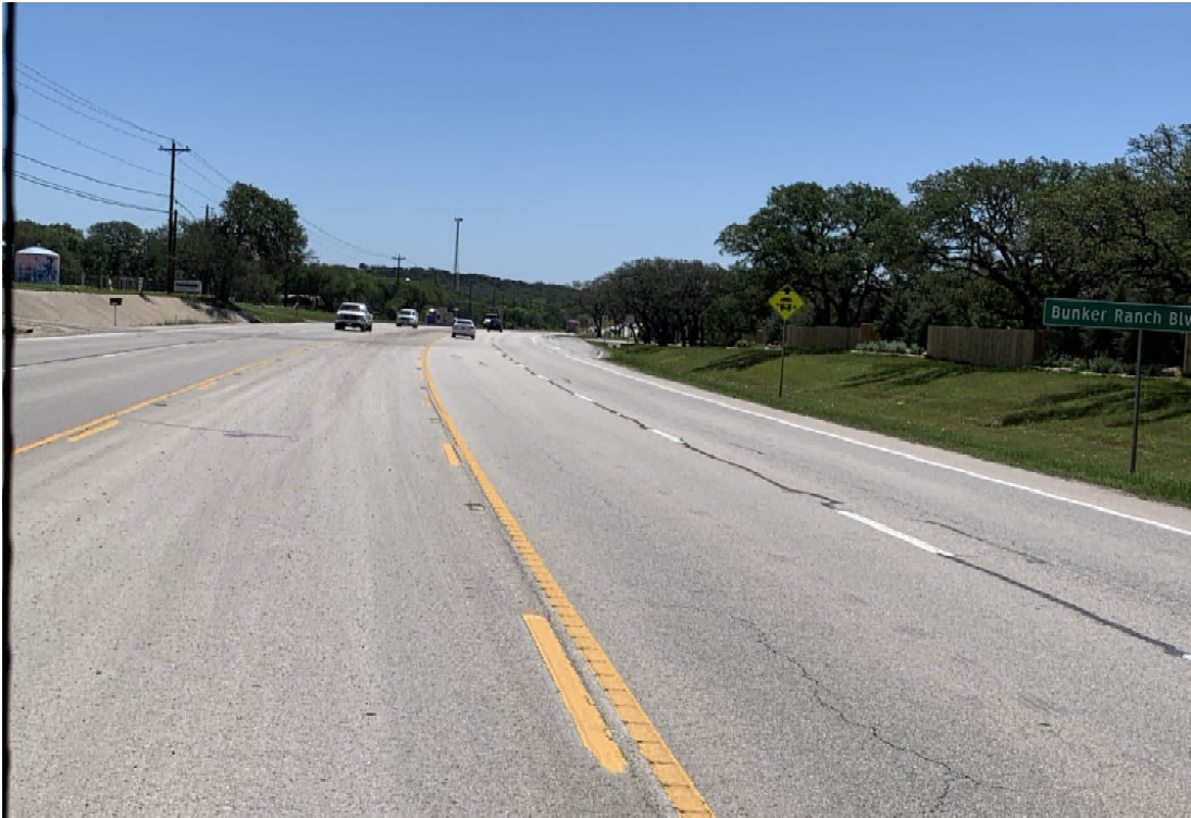
Eastbound US 290 Approach
