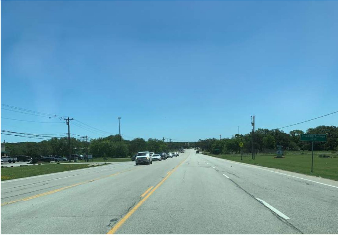
Eastbound US 290 Approach
