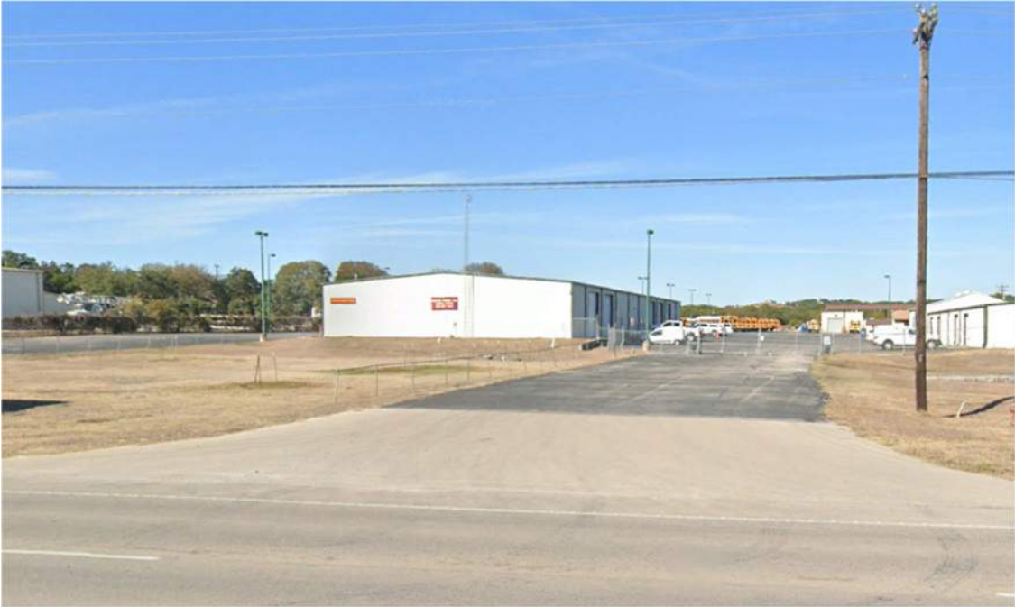
Looking at Southbound DSISD Driveway
