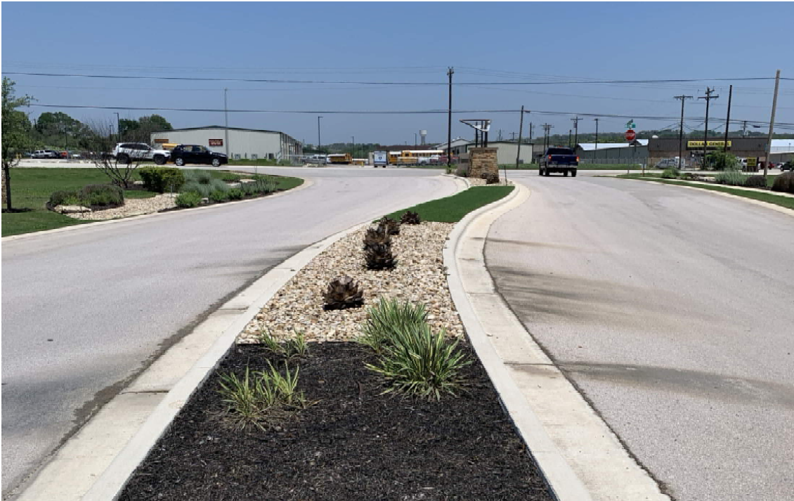
Northbound Arrowhead Ranch Boulevard Approach
