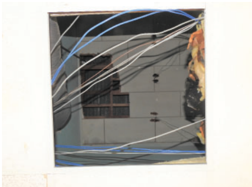
Figure 3.42: Original ceiling panel finish found above dropped ceiling
