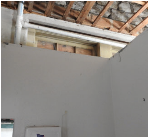
Figure 3.17: Original window boarded-over on exterior with restroom furr-out wall on interior
