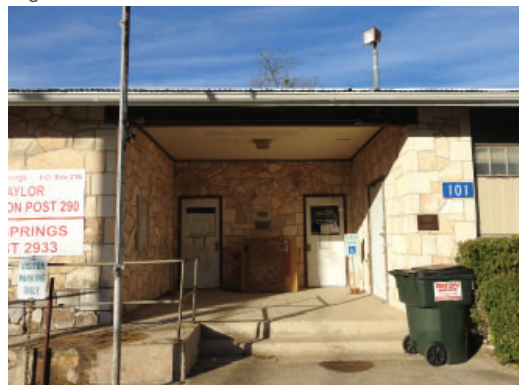
Figure 3.6: Recessed opening at the east elevation
