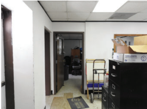
Figure 3.40: Occupied space. Note non-original VCT tile flooring, dropped ACT ceiling, and furred-out wall
