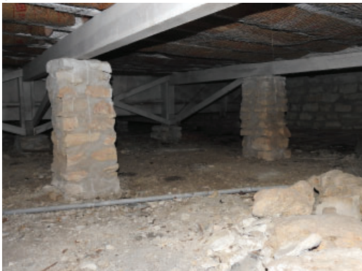
Figure 3.2: Limestone masonry pier and wood beam structure
