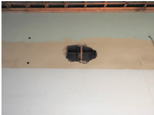
Figure 3.34: Original interior wall. Note three paint colors, signifying the addition of two dropped ceilings
