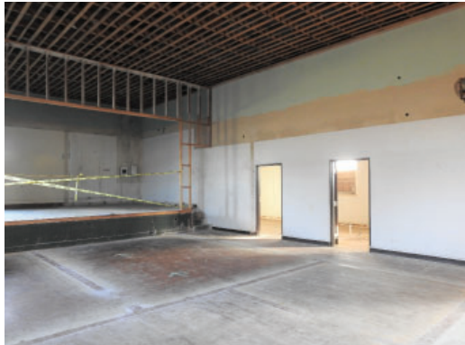
Figure 3.33: Main auditorium space. Note original wood flooring and load bearing interior wall. Stage to the left
