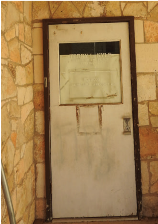
Figure 3.22: One of two main entry doors, non-original door in original opening
