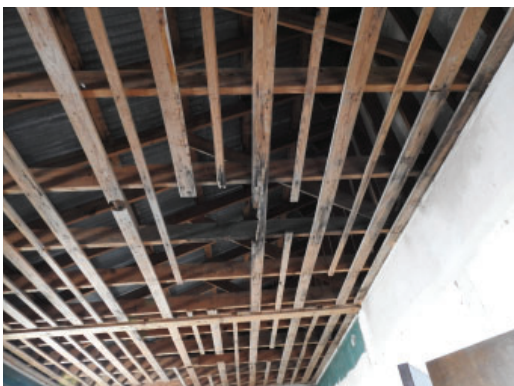
Figure 3.12: Wood trusses visible through ceiling
