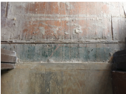
Figure 3.39: Threshold between remodeled space and main auditorium
