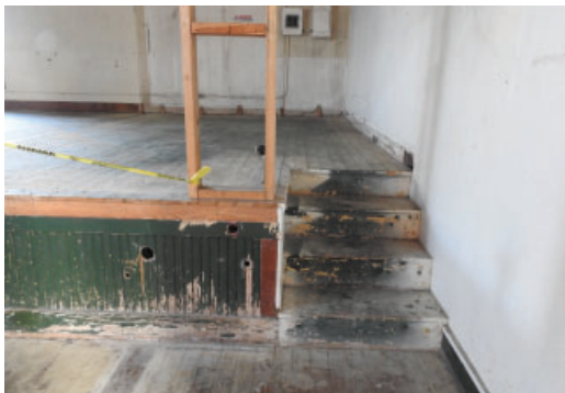
Figure 3.47: Stairs to stage. Note wood beadboard proscenium
