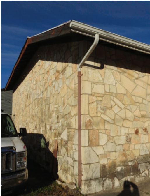
Figure 3.31: Single metal gutter at southeast corner
