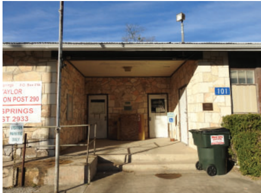
Figure 3.27: Recessed, covered entrance on east elevation
