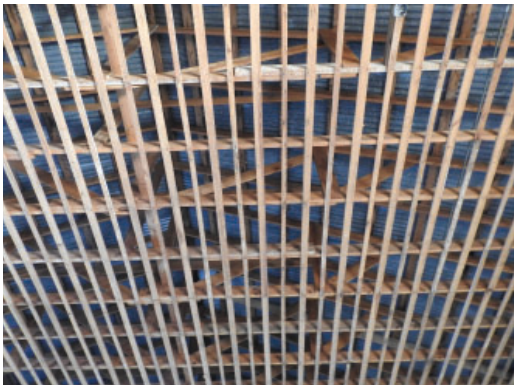
Figure 3.11: Wood trusses visible through ceiling
