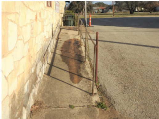
Figure 3.53: Ramp leading to concrete platform
