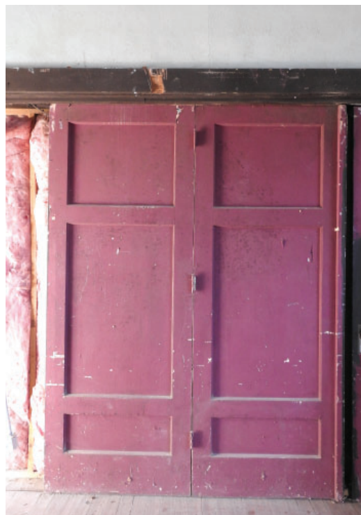
Figure 3.44: Three panel wood doors with original hardware
