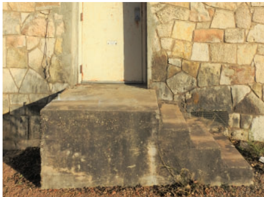
Figure 3.54: Concrete steps up to entrance landing
