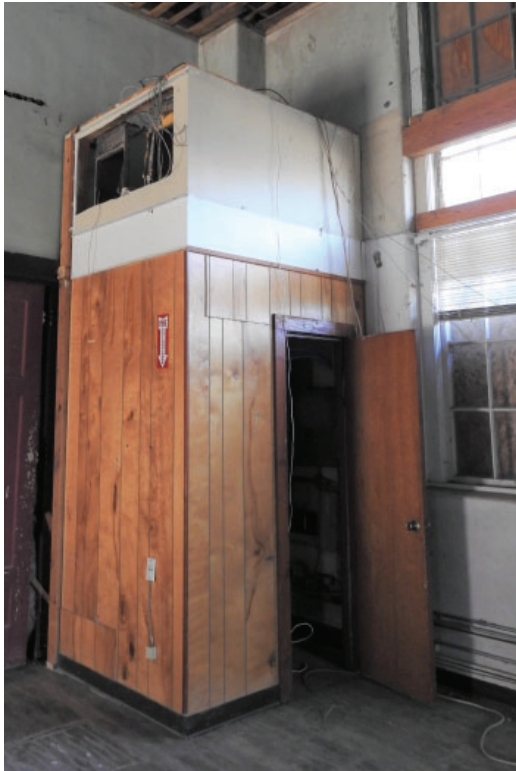
Figure 3.37: Non-original mechanical room addition. Note original chimney floor behind
