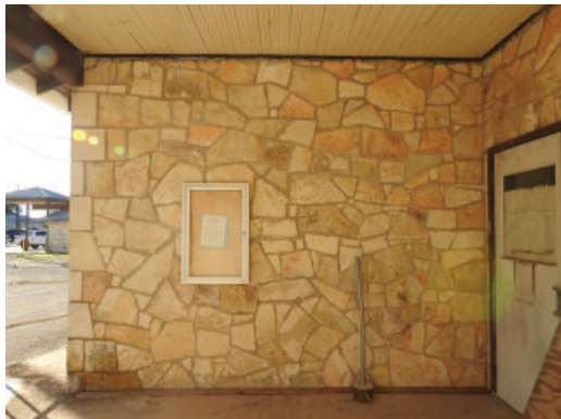
Figure 3.28: South face of recessed, covered entrance
