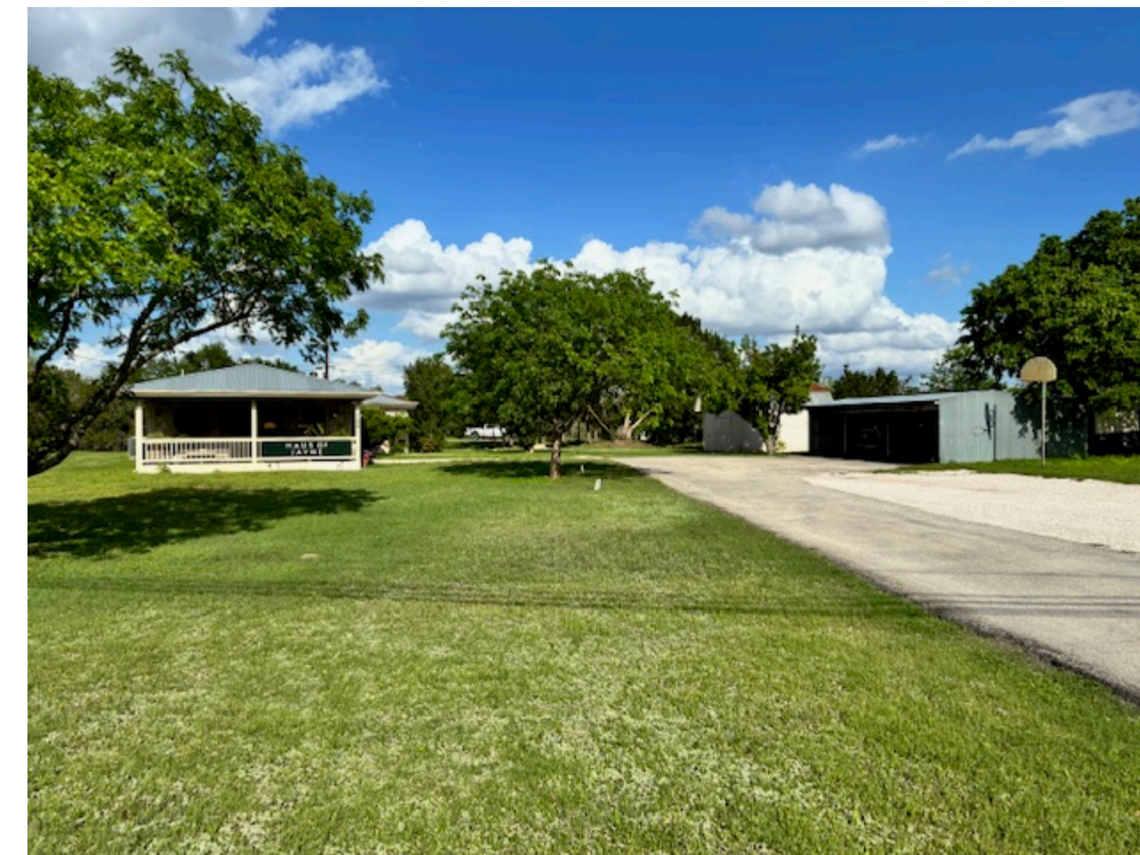
Subject Property - Project behind Carport Building
