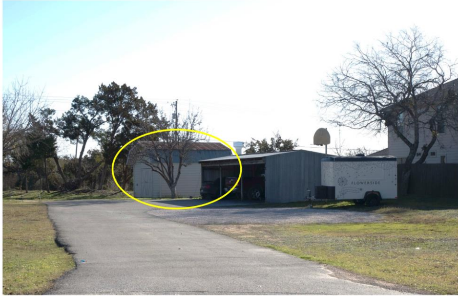
766 Old Fitzhugh Shed: “Current Conditions, view from Old Fitzhugh Rd”. Historic Survey images, 2024
