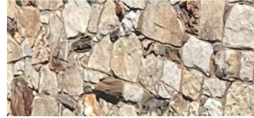
EXISTING MASONRY TO REMAIN
