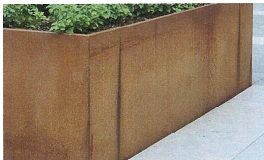
1. Corten Steel Frame
