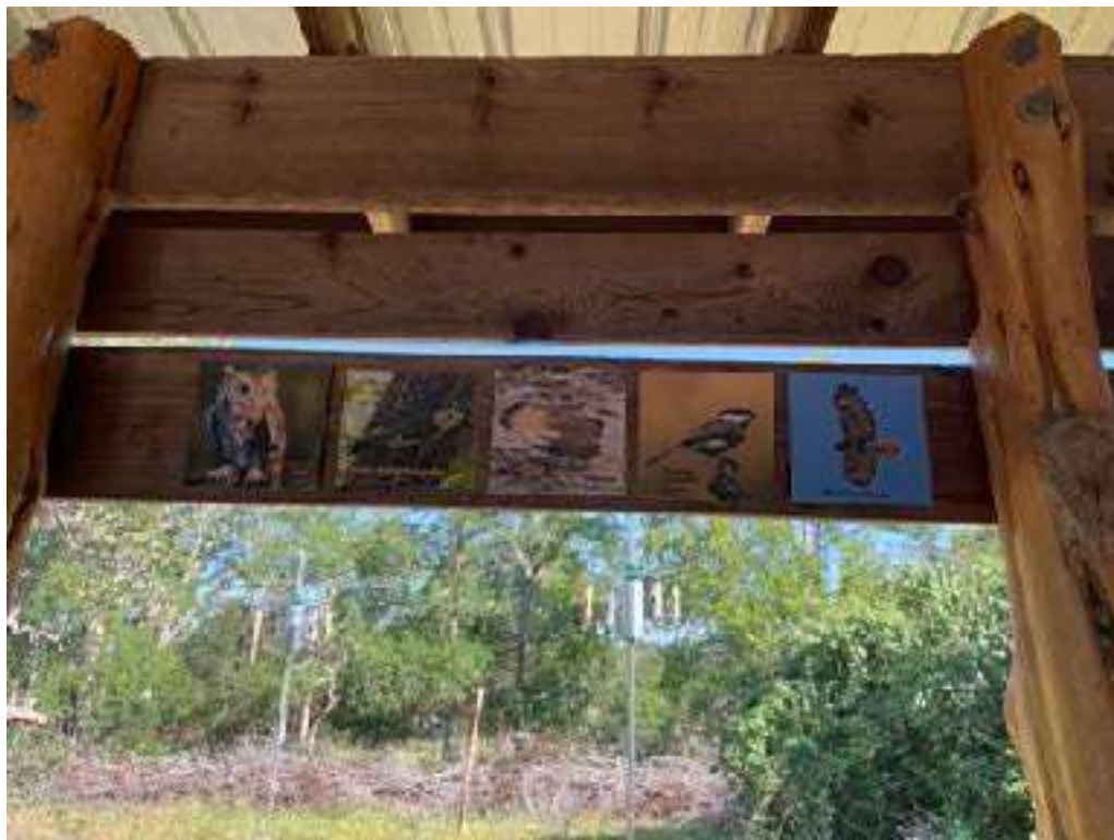
A view of 6" signs on 8" boards near roof of blind - north side.
