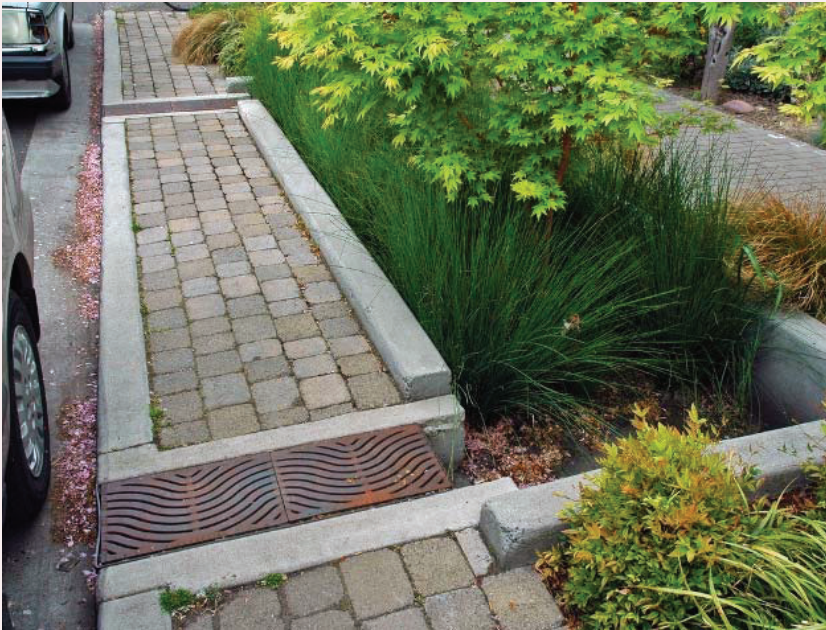
STRUCTURED RAIN GARDEN
