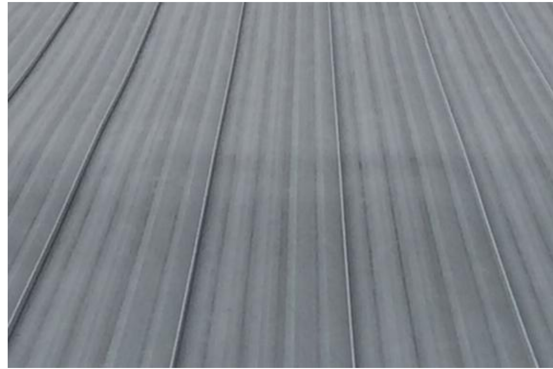
Pre-Weathered Galvalume Standing Seam Roofing Panels installed on new additions
