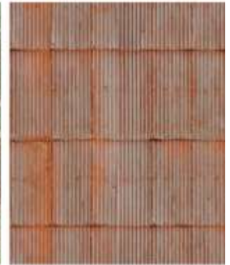
Reclaimed metal panel from existing wood shed
