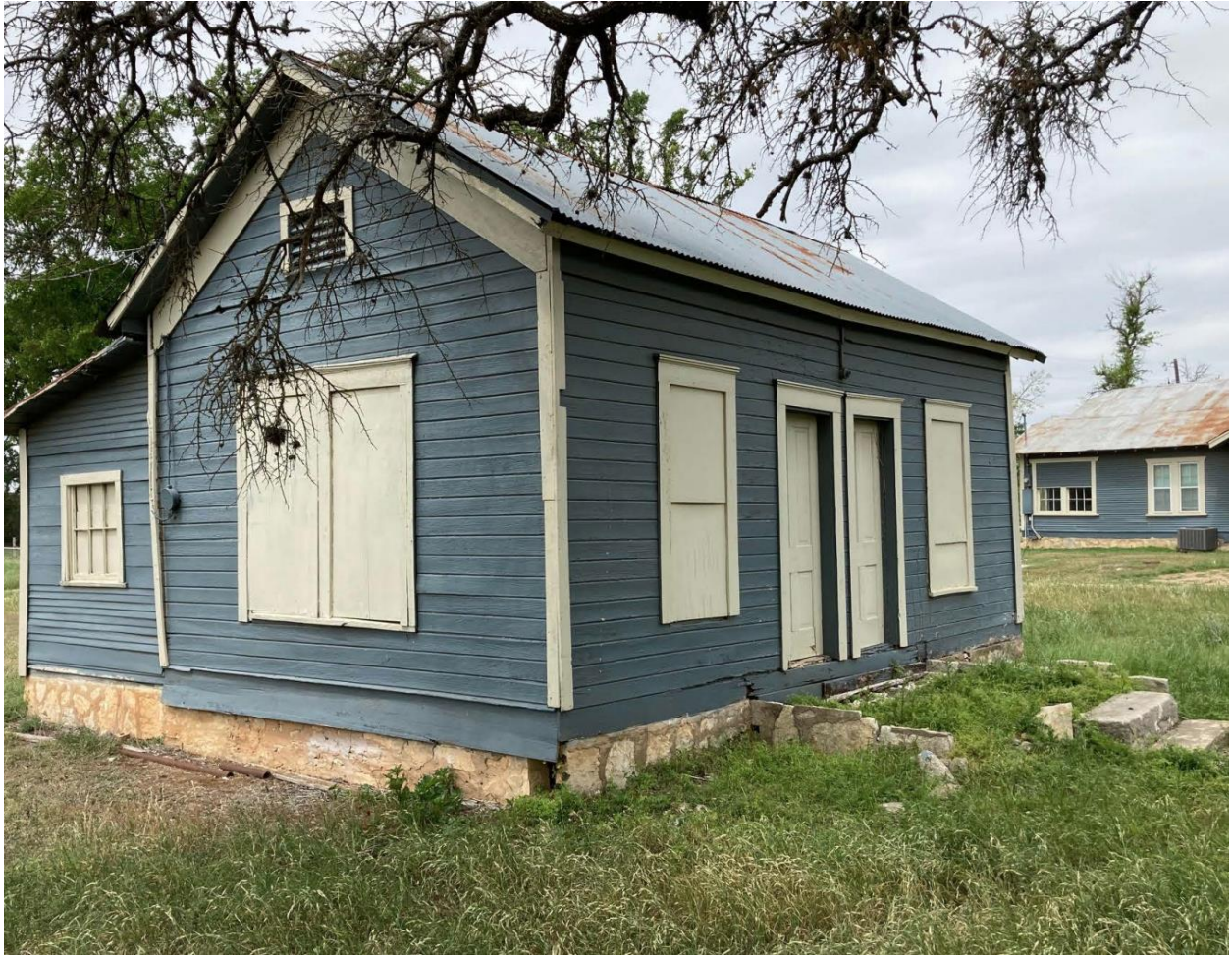
215 Old Fitzhugh Road: "Current Condition". 2024
