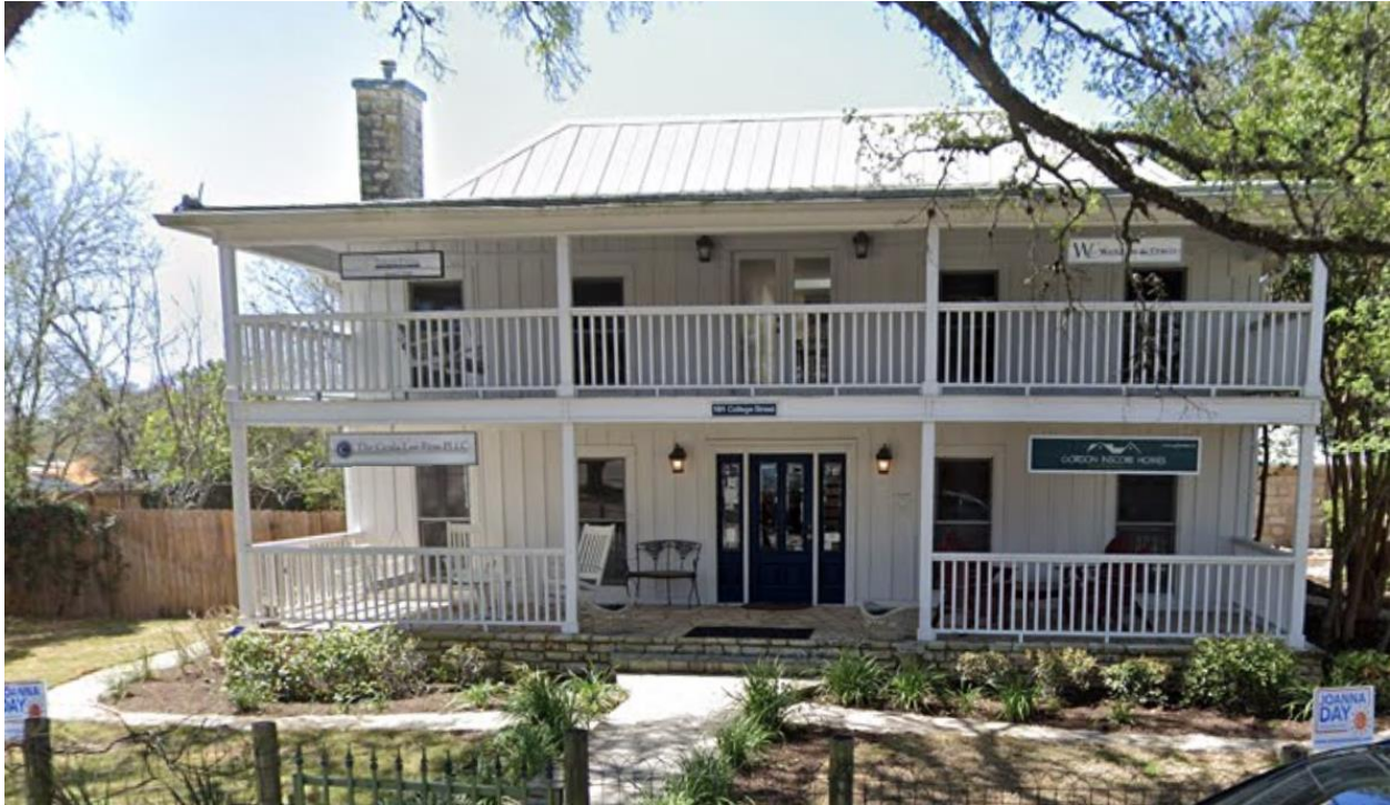
101 College St: “Current Condition”. Images from Google Maps, 2019.
