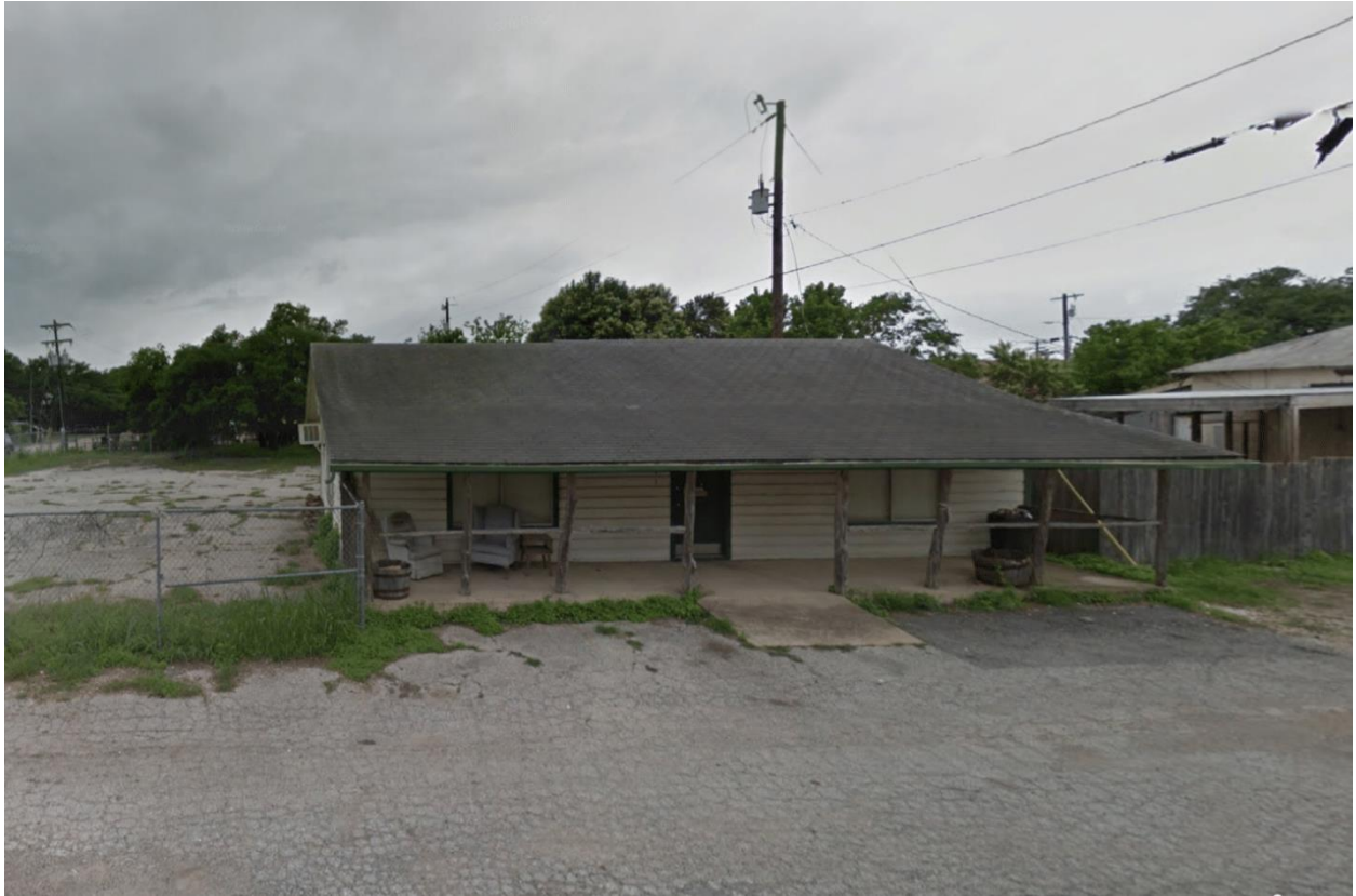
101 San Marcos St: “Current Condition”. Images from Google Maps, 2023.
