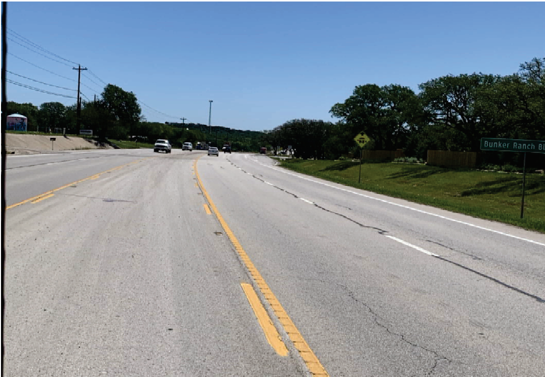
Eastbound US 290 Approach
