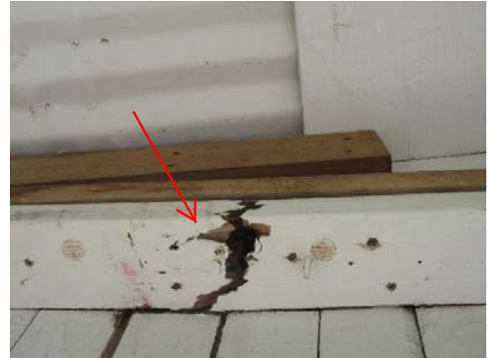
Masonry cracking: The masonry at the front porch is cracking and shows signs of general settlement.
