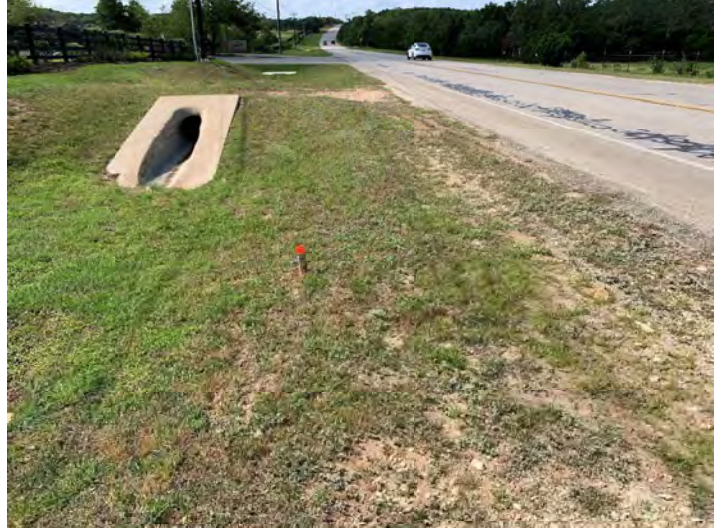
Photo 6: Existing pipe end treatment proximity to Shared Use Path extension Gus Drive.
