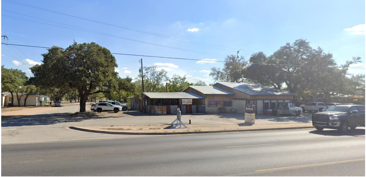
301 W US 290: “Current Condition, view from US 290”. Images from Google Maps, 2023.
