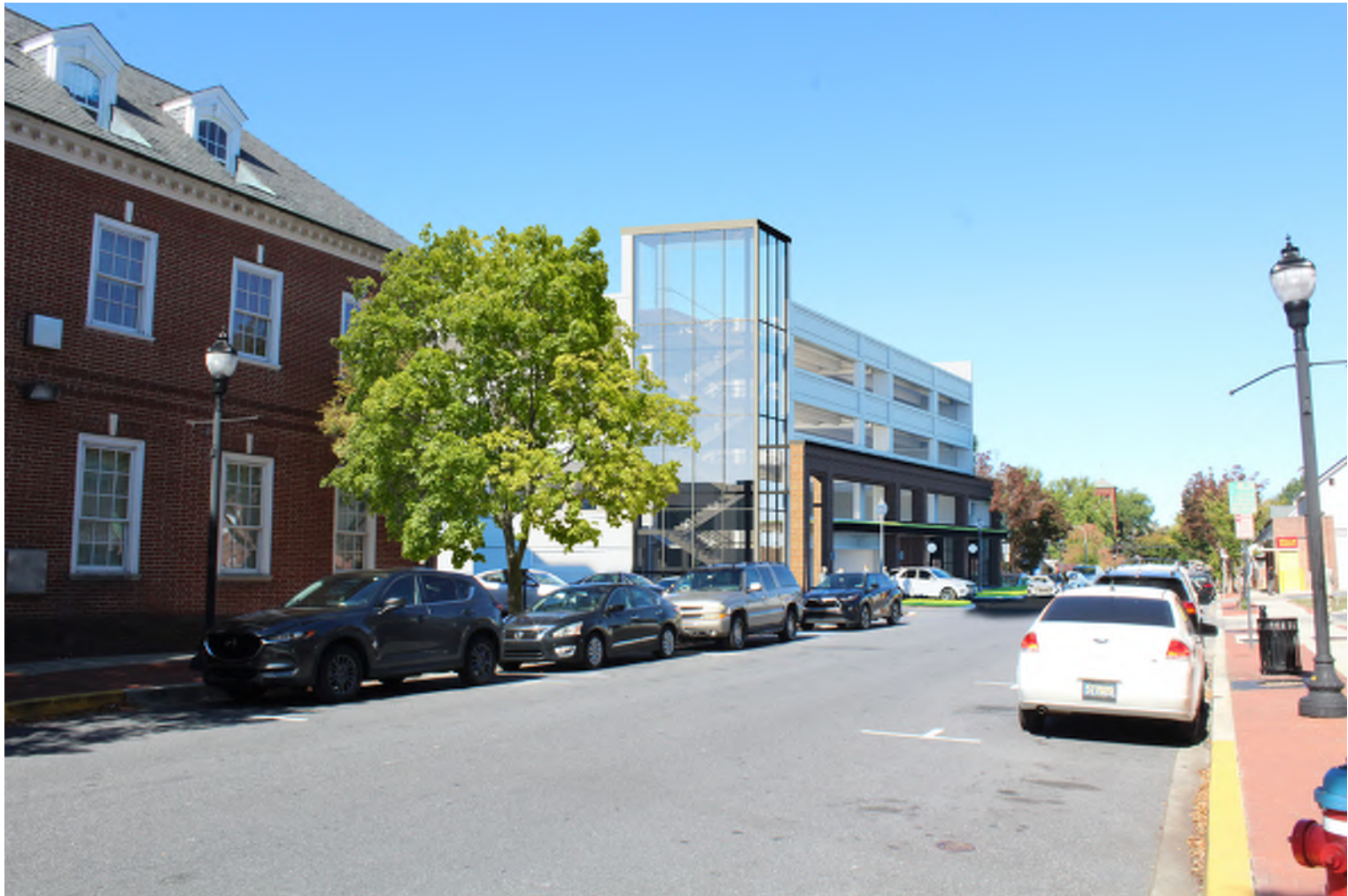
1: VIEW FACING NORTH FROM S BRADFORD STREET
