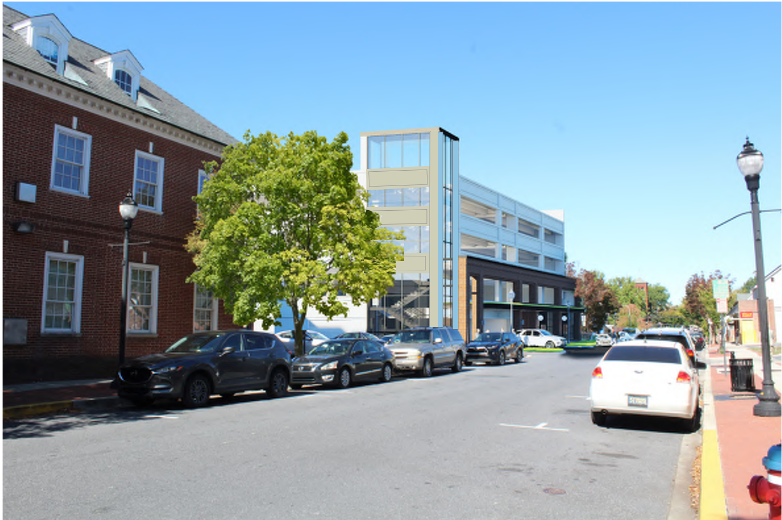
1: VIEW FACING NORTH FROM S BRADFORD STREET
