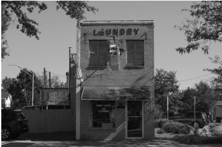
C: GOVERNORS AVENUE, NEIGHBORING BUILDING
