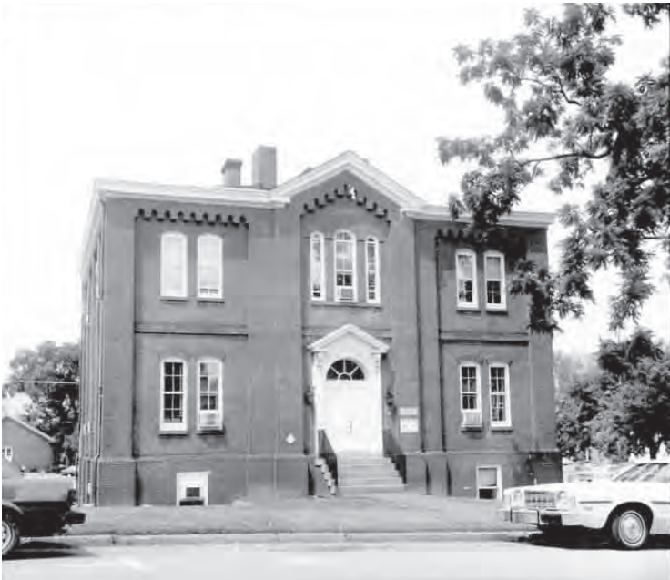
Figure 3.1.12 Old County Building South Façade (1986)
