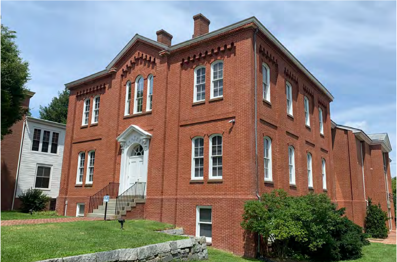
Figure 2.3.2 Existing View of The Biggs Museum - Old County Building Portion of the Building
