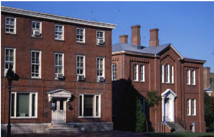
Figure 3.1.13 Old County Building Southwest View (1998)
