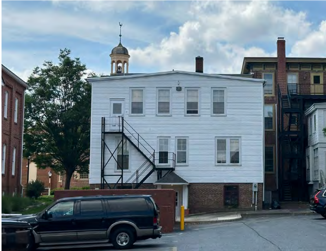
Figure 2.3.6 Existing View of 21 The Green North Elevation
