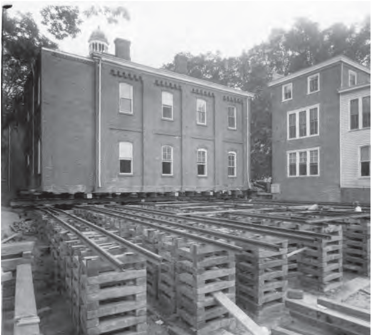
Figure 3.15 Old County Building Relocation (1932)
