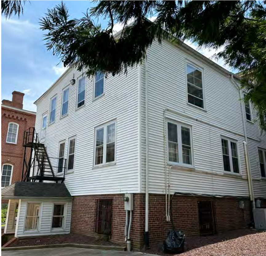
Figure 2.3.7 Existing View of 21 The Green Northwest View
