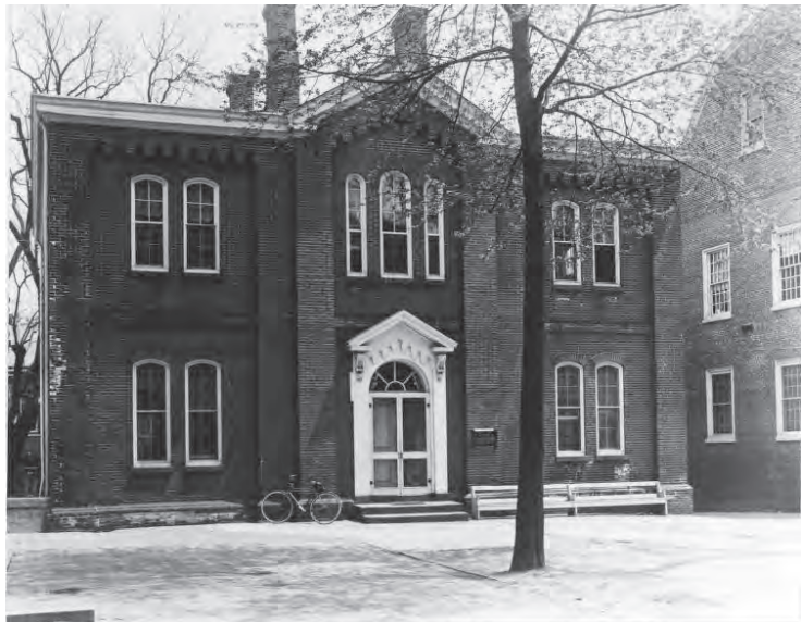
Figure 3.1.4 Kent County Building (1923) Prior to its Relocation
