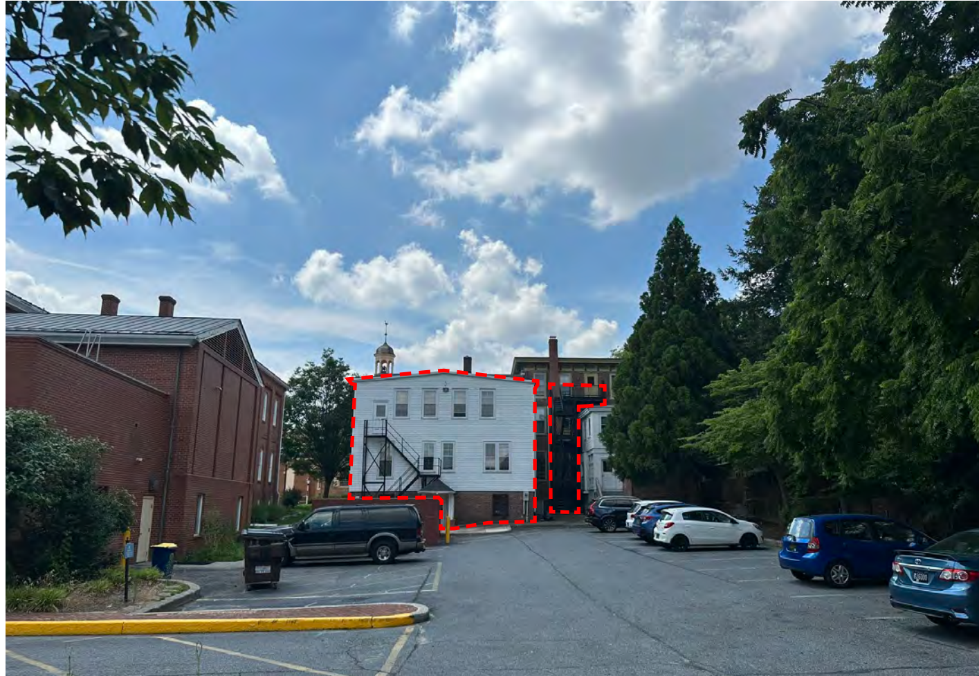
Figure 4.2.10 Existing View from Northern Edge of Existing Parking Lot (Red Outline Denoting Proposed Selective Removal)
