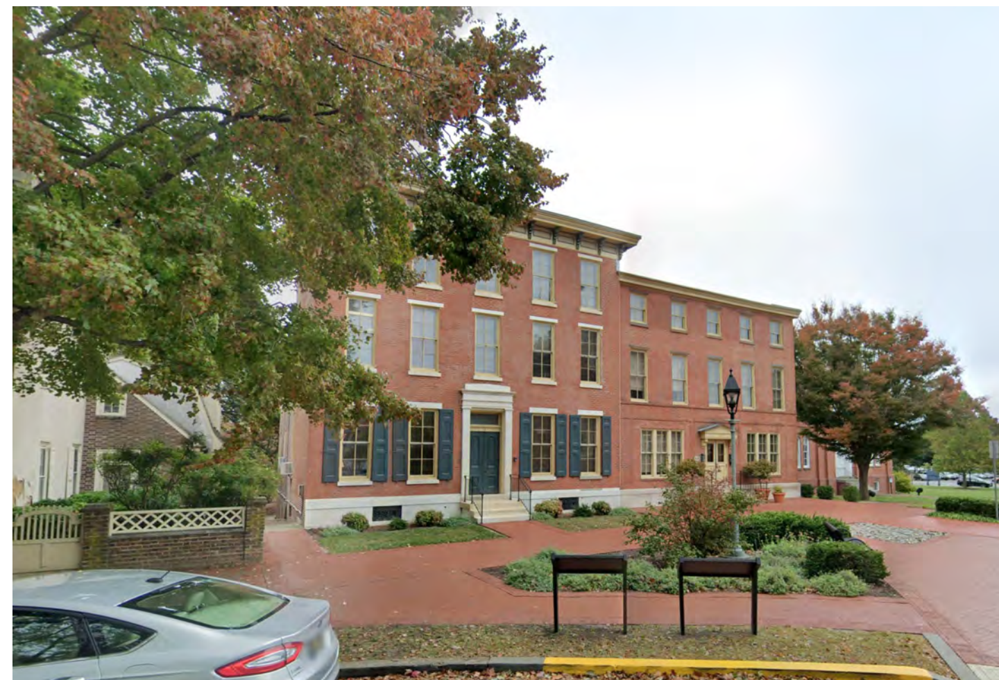
Figure 4.2.9 Existing South View of 15 and 21 The Green (Showing No Impact from The Green of Proposed Selective Removal)
