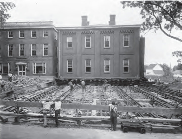
Figure 3.16 Old County Building Relocation (1932)
