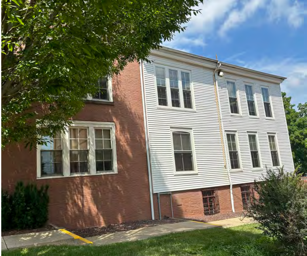
Figure 2.3.4 Existing View of 21 The Green East Elevation with Referenced Rear Addition Recommended for Removal
