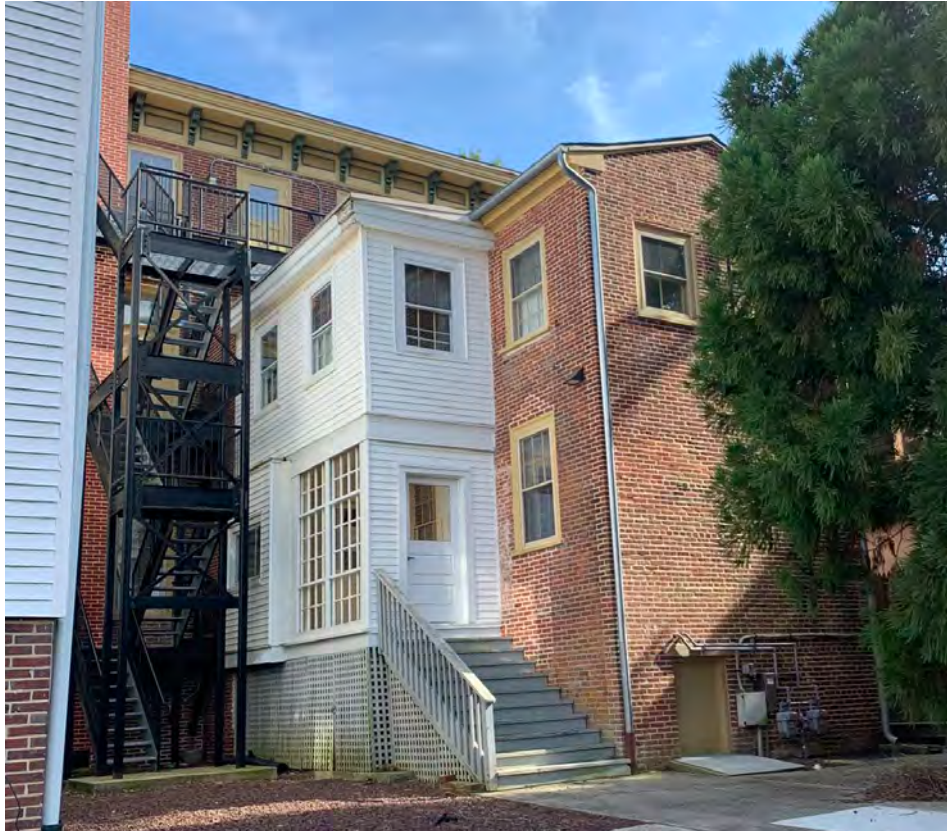
Figure 2.3.8 Existing View of 15 The Green North Elevation
