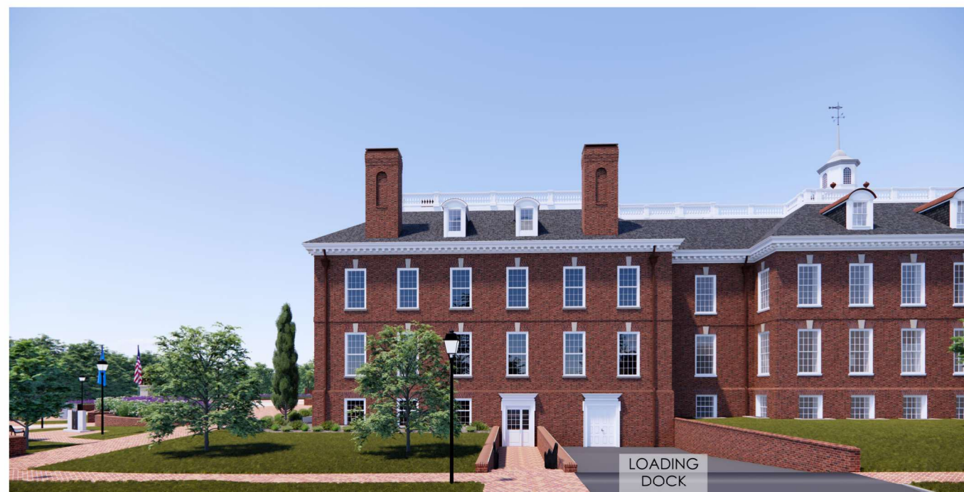
7 - VIEW OF LOADING DOCK ON MLK JR BLVD N
