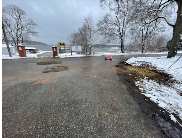
Wall Street (Douglas) Water Leak March 2023
