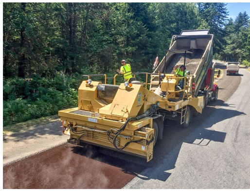
• Chip Sealing
