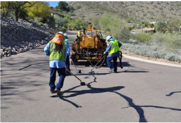
• Crack sealing
