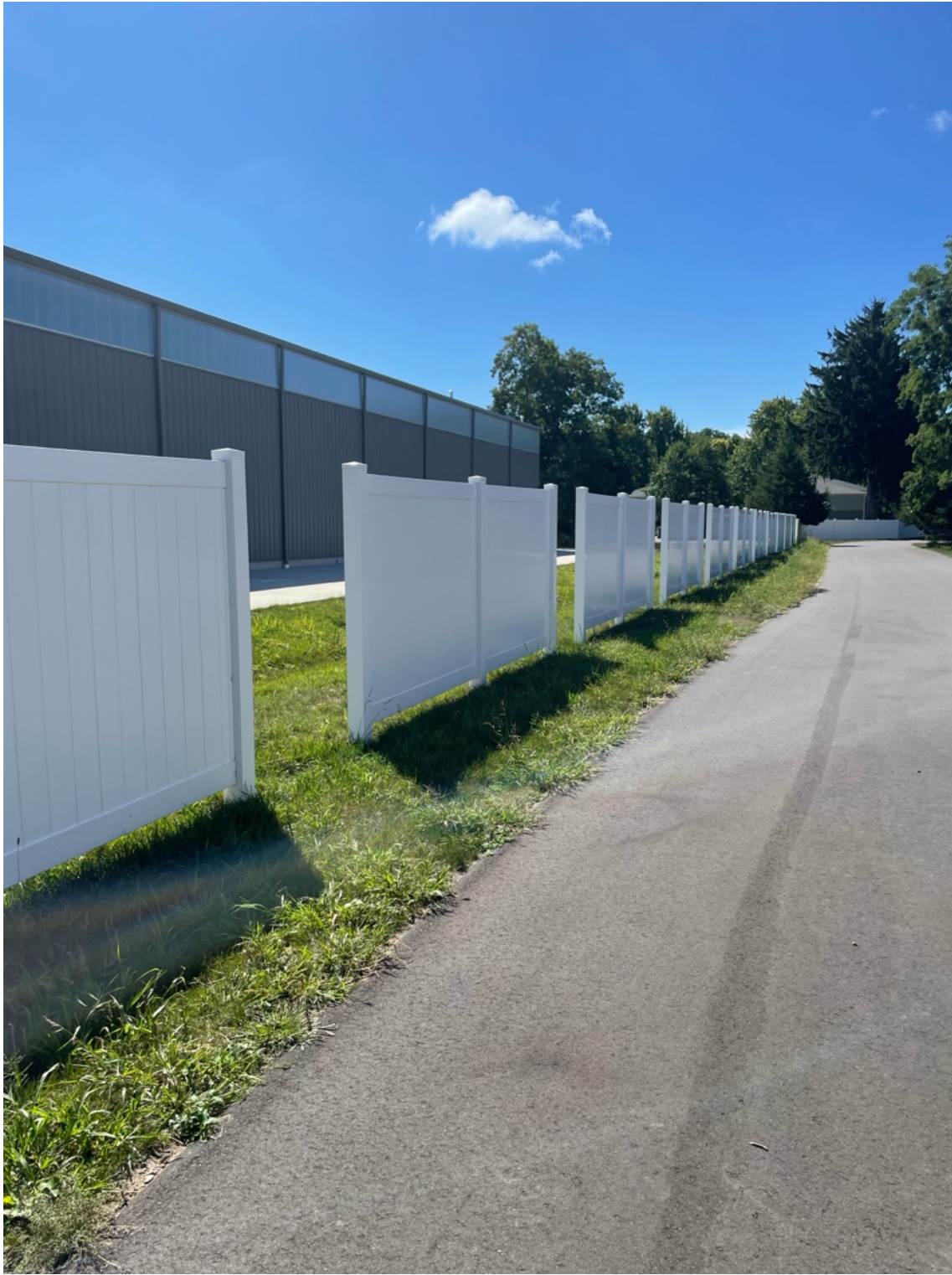
4.) Post Construction: Back of building Showing Current Fence Panels South View
