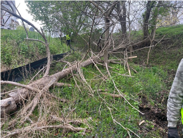
Roadside ditch then drains north onto Swingbridge and Milauckas property. No swale appears to be constructed and notice silt fence east of where swale disturbance would have been.
