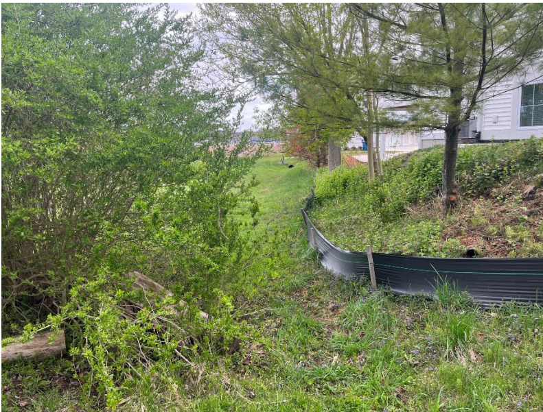
Roadside ditch then drains north onto Swingbridge and Milauckas property. No swale appears to be constructed and notice silt fence east of where swale disturbance would have been.
