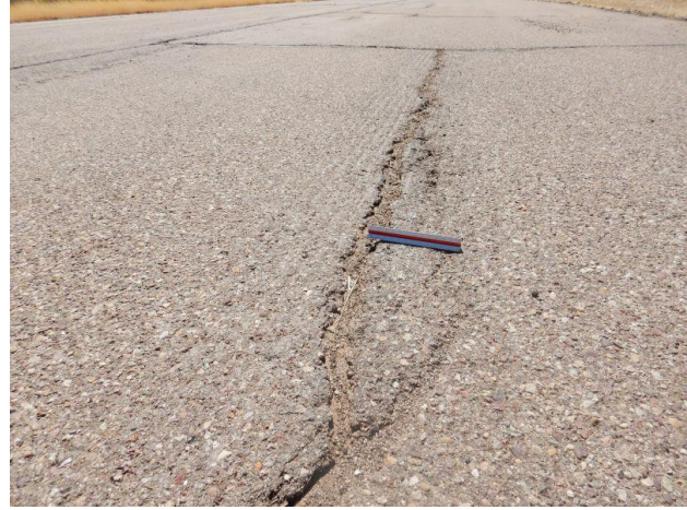
Photo 2.2d – Asphalt Swelling
