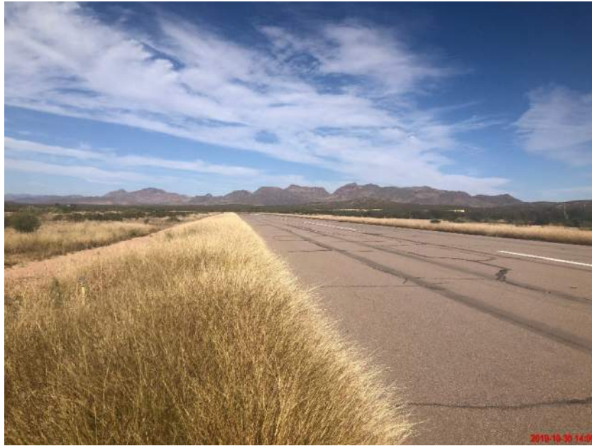
View from the project limits looking northeast along Runway 03-21.
