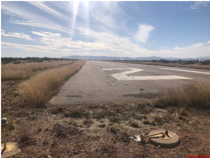
View from the northeast corner of the project limits looking southwest along Runway 03-21.
