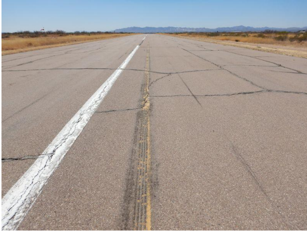
Photo 2.2c – Existing Runway Pavement
