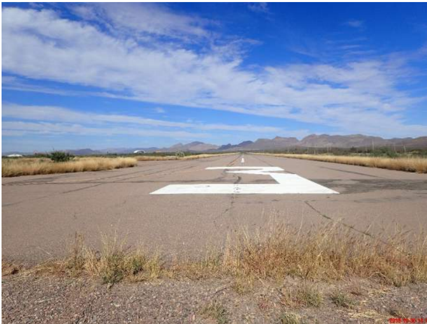
View from the southwestern project limits looking northeast along Runway 03-21.
