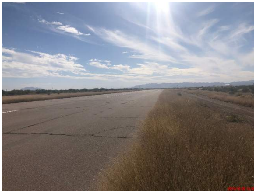
View from the project limits looking southwest along Runway 03-21.
