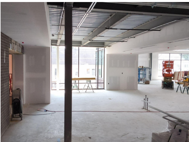
Addition looking south
