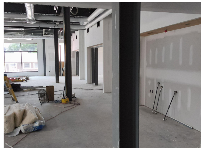
Addition looking west along community room
