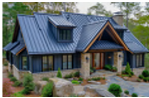
METAL ROOF STANDING SEAM [M1]
