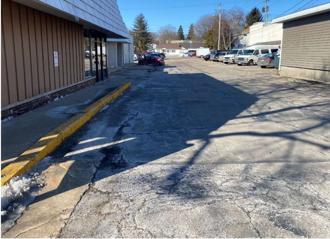
Photo 5: View of north parking lot from Main Street.
